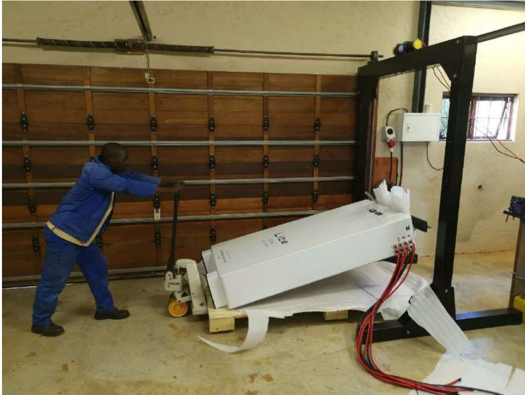
Fig 3.5 Site Assembled Gantry with Electric Hoist
